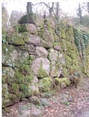
A drystone wall in Manor Brook showing the large stone sizes used.
