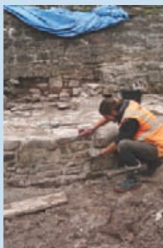
Above: Lime mortaring
