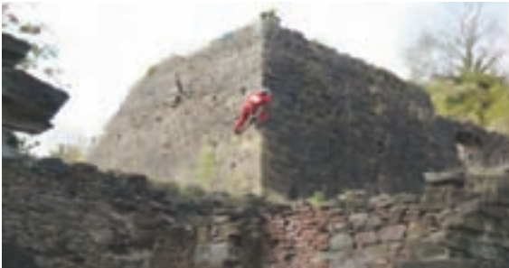
Rope access survey of main furnace structure
